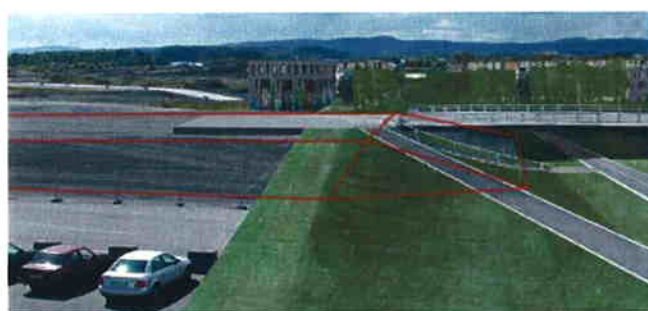
Figure 5 Use of PAH-contaminated soil in road construction at Fornebu, present situation (top) and future situation (bottom)
