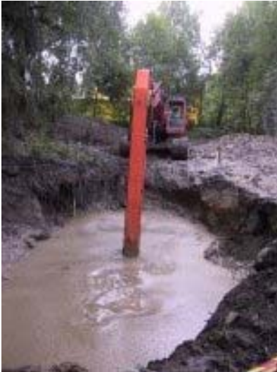
Picture 1. Biopolymer slurry construction method
